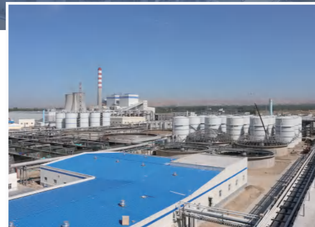
伊犁川宁生物技术有限公司二期废水治理EPC项目 EPC project for second-phase waste water treatment of Yili Chuanning Biotechnology Co., Ltd.
