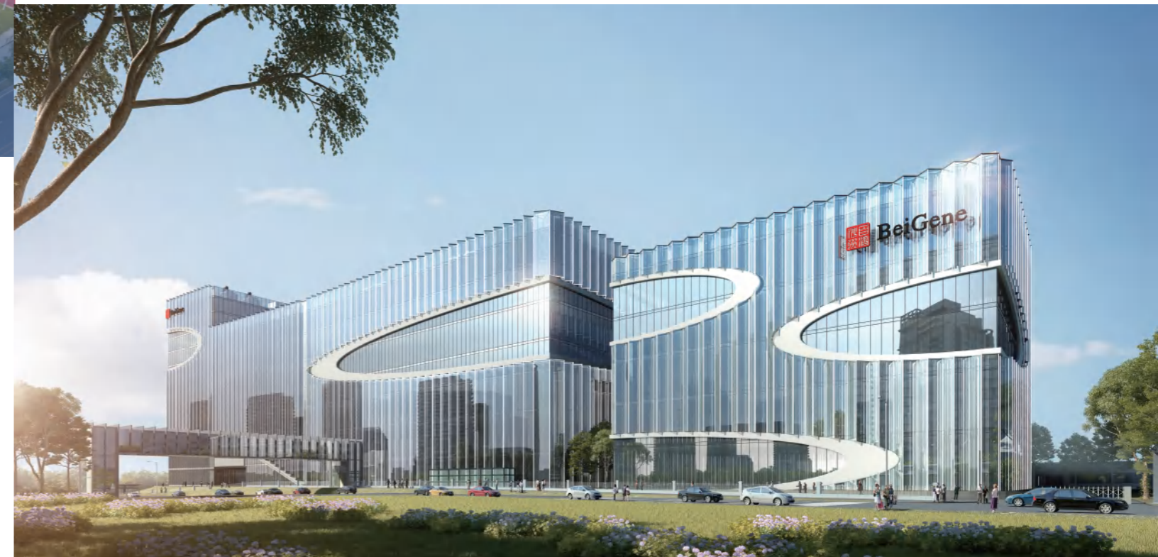
广州百济神州生物制药有限公司ADC及DS4生产车间机电安装及洁净装修工程 ADC and DS4 production workshop mechanical and electrical installation and clean decoration works of Guangzhou BeiGene Biopharmaceutical Co., Ltd.
